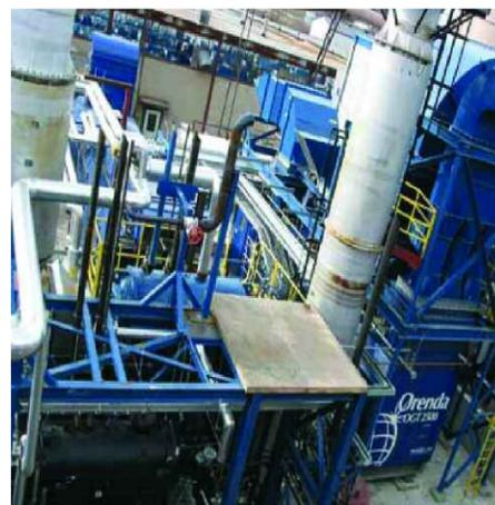
Figure 3: The Orenda OGT 2500 Turbo-generator installation at the Dynamotive West Lorne co-gen plant.
