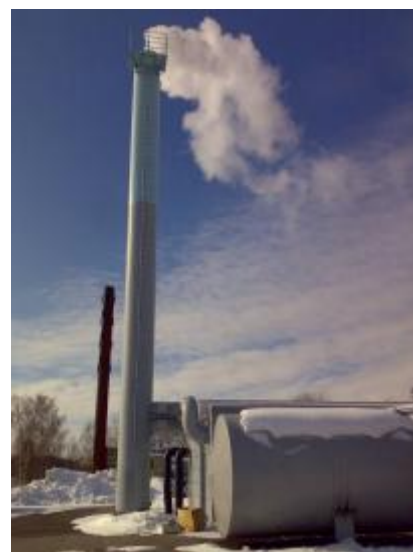
Figure 2: Fortum's Masala site burning bio-oil. The light fuel oil tank is at the front
