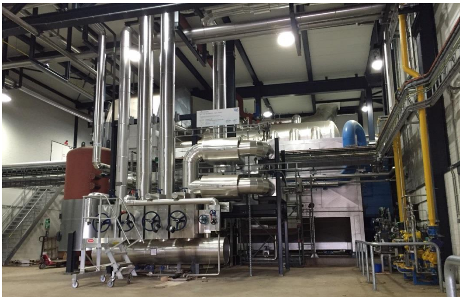
Figure 2: FPBO fuelled process steam boiler at FrieslandCampina in Borculo, the Netherlands. Up to 4 t/hr of FPBO is co-fired with natural gas". Picture Empyro/FrieslandCampina
