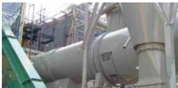
Figure 2: feedstock preparation under construction.
