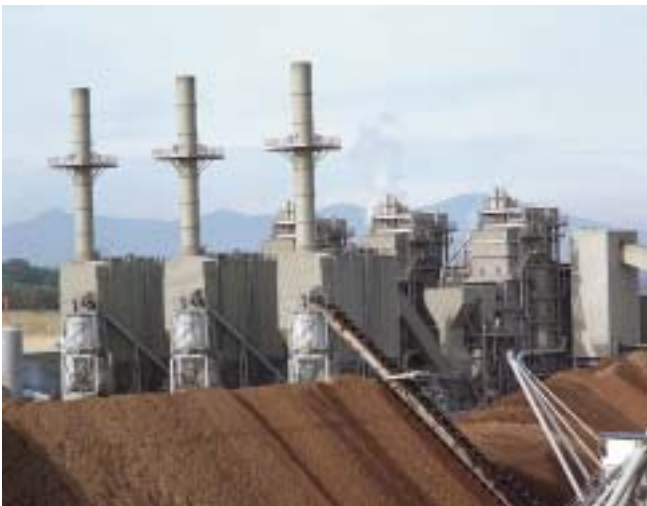
Figure 1: Shasta Power Plant, Anderson, CA (Warren Gretz-NREL).
