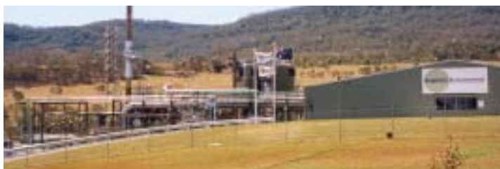
Figure 1: Brightstar Environmental's SWERF gasification plant near Wollongong, Australia.
