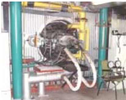
Figure 1: Co-combustion of bio-oil produced by BTG Biomass Technology Group in Electrabel's 350 MWe gas-fired power station in Harculo, The Netherlands. Photograph of the burner front side showing the pressurized bio-oil lines including the atomization pressure indicators. Reproduction of the photographs is subject to permission by Electrabel and BTG.
