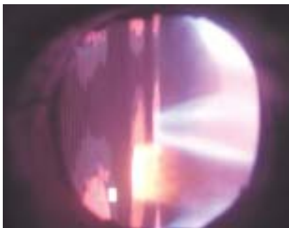
Figure 2: Co-combustion of bio-oil produced by BTG Biomass Technology Group in Electrabel's 350 MWe gas-fired power station in Harculo, The Netherlands. Photograph of the boiler room side of the bio-oil burner and its (orange) flame. Eight other burners in the boilers house (55 MWth each) were fired on natural gas (blue flame). Reproduction of the photographs is subject to permission by Electrabel and BTG.
