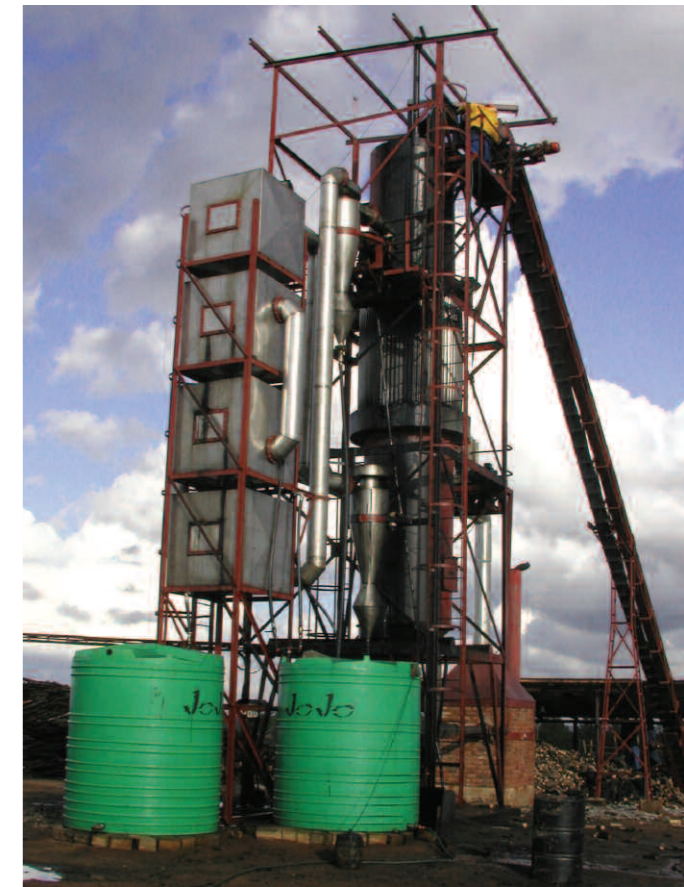
Figure 2: RWC's Slow Pyrolysis facility
