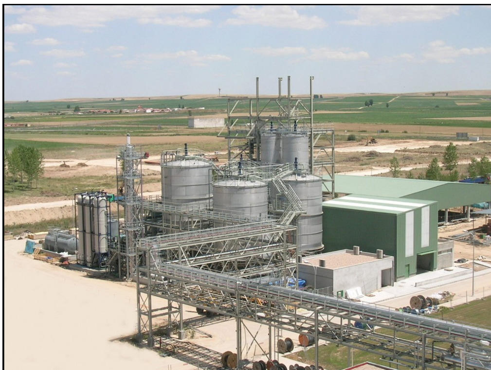
Figure 2 Abengoa Bioenergy New Technologies (ABNT) pilot plant for processing straw into ethanol at Salamanca in Spain
