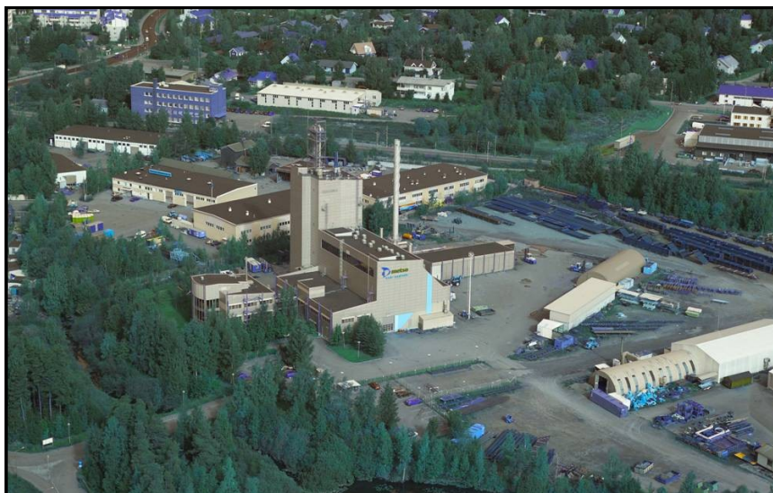
Figure 1; A 2 MW fuel fast pyrolysis unit has been integrated with Metso's 4 MWth circulating fluidized bed boiler, located at Metso's R&D Centre in Tampere
