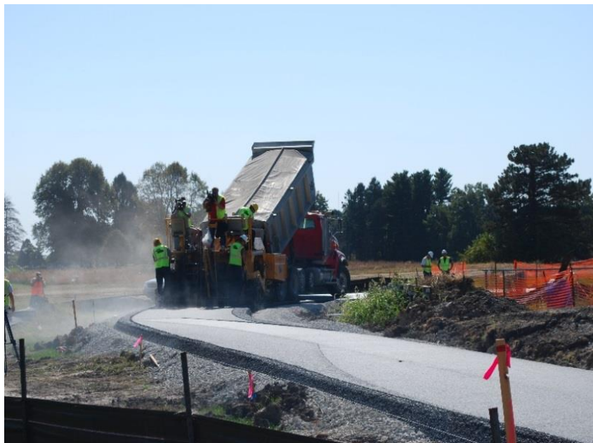
Fig. 3 – Paving Waveland Bike Trail, Des Moines, IA with a mixture of petroleum-based asphalt and phenolic oil.
