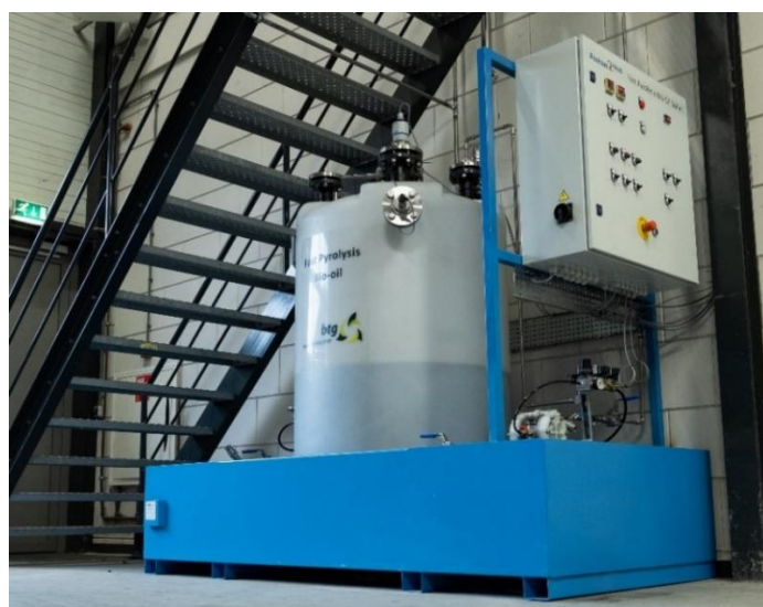
Fig. 5: FPBO fuel storage and feeding system.
