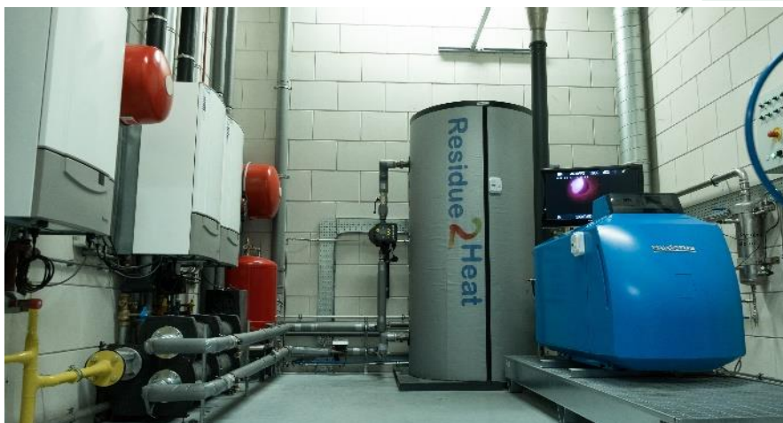
Fig. 4: FPBO boiler system (right side) integrated with the existing natural gas fired boilers (left side)
