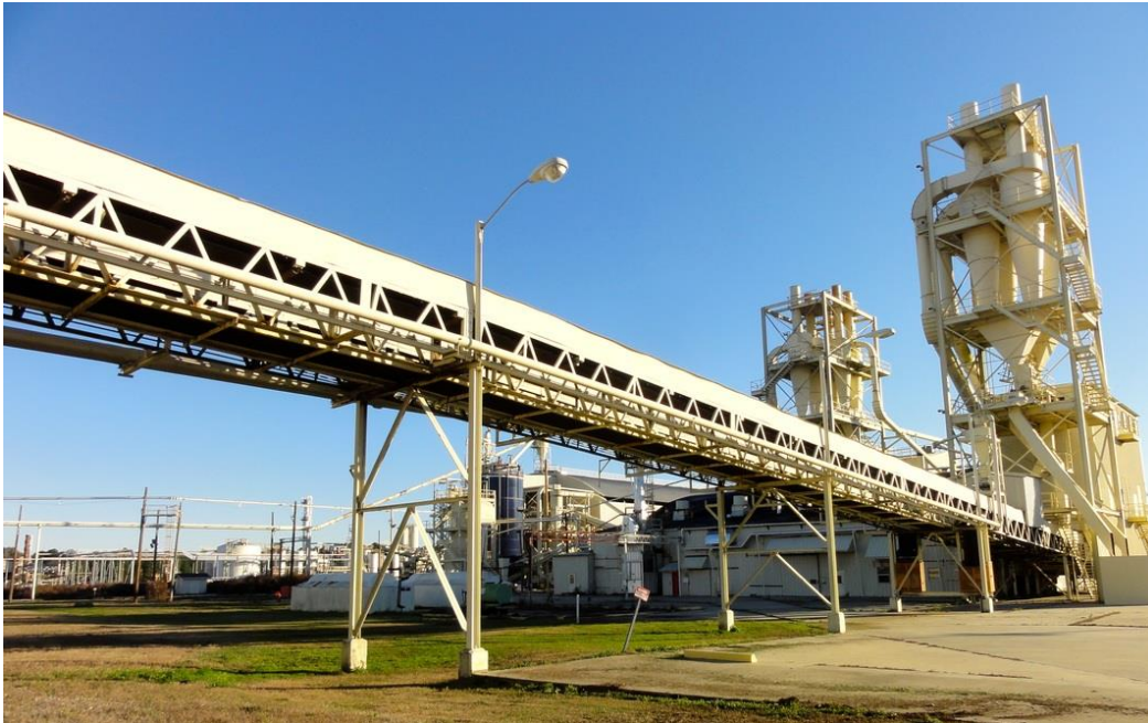
Roseberg Forest Product's particle board mill in Dooley County, Georgia. This mill is the proposed site of a Rapid Thermal Processing (RTP) plant proposed by Ensyn Development Partners.
