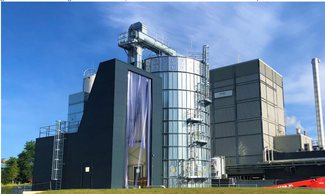
Fig. 5 B : New biomass storage; storage capacity 1 – 2 days
