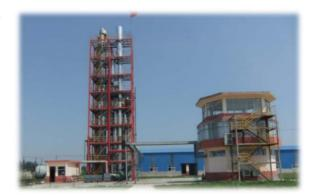
The demonstration plant at Dali County in China utilises downdraft circulating fluidised bed fast pyrolysis technology. The facility processes 1-3 tonnes/hour of rice husks producing pyrolysis oil as the major product, as well as char and non-condensable gas. Though the plant is still operational, it is not used on a daily basis.
