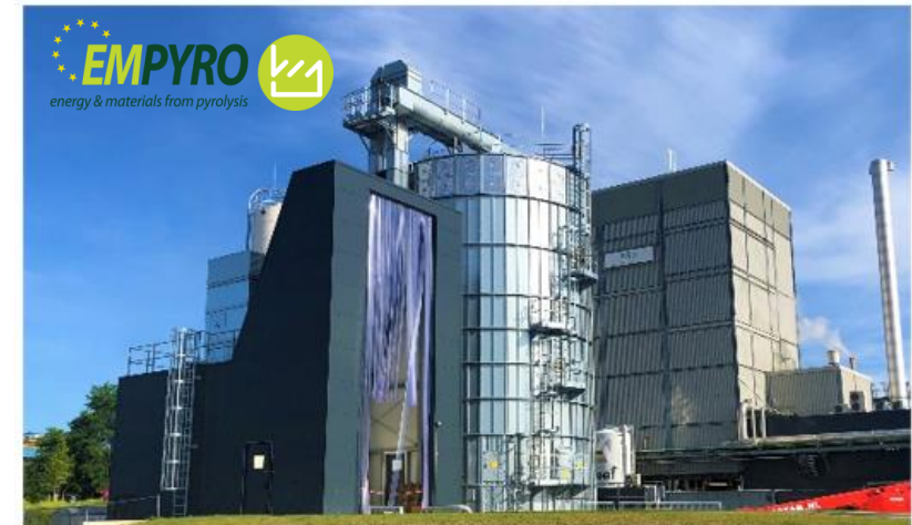
Empyro: 25MW Fast pyrolysis plant in NL
